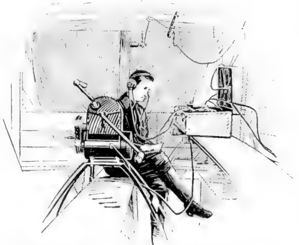
Interior view showing the apparatus in working order
